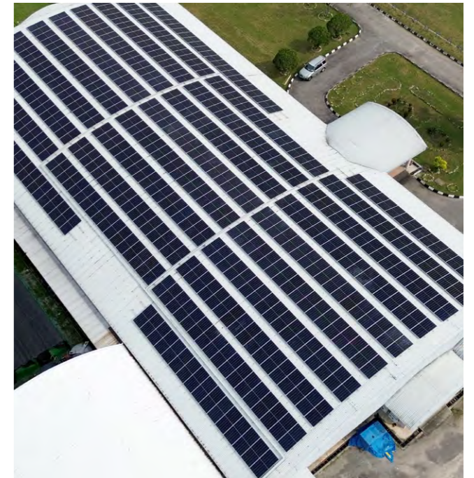
» Rooftop solar PV system under Net Energy Metering (NEM) scheme with Power Generation of 342,669 kWh/year installed at SD Guthrie's R&D centre at Banting, Selangor, Malaysia.
